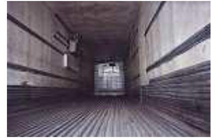
TUNNEL MOUNTED RAD-21 CANSCAN
